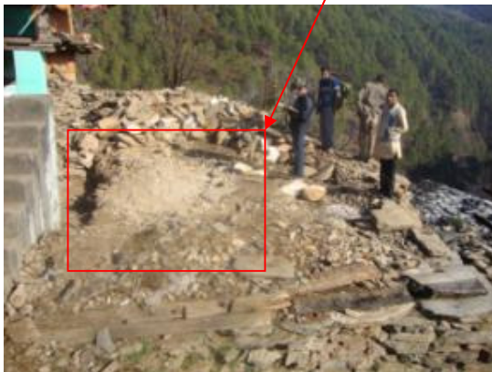
A Side view of the site from West direction.
