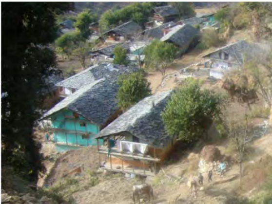
A far view of the proposed site from West direction.
