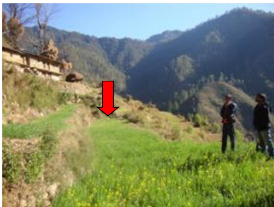
A side view of the construction site.
