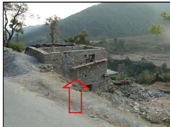
Back side view of the site
