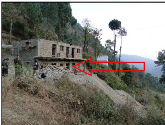
under construction house on the propose site
