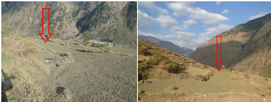
Valley side and side view of the site
