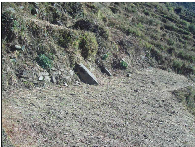
Side view of the proposed site for construction
