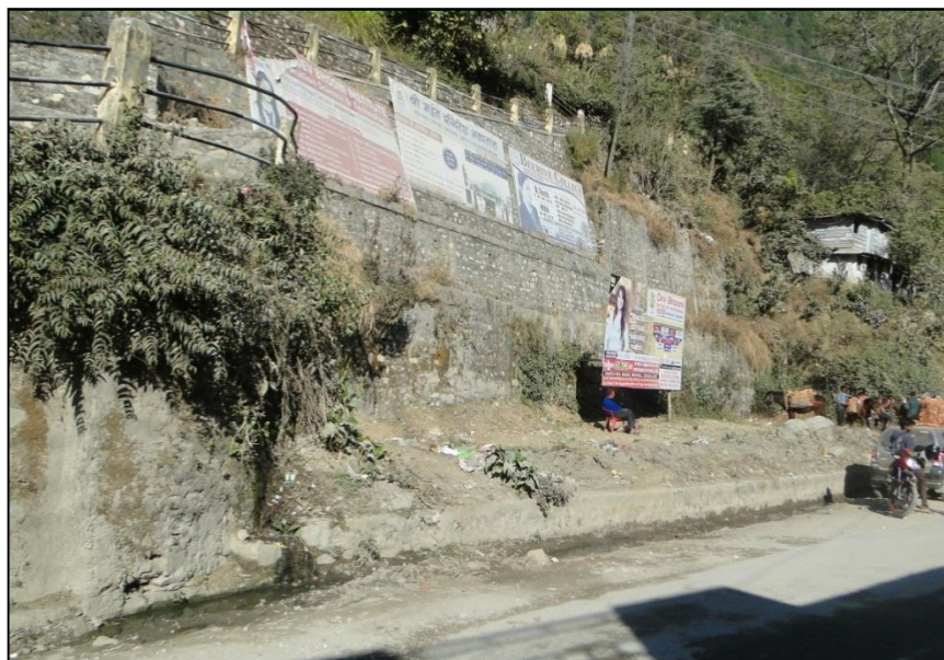
Hillside view of the proposed site for construction
