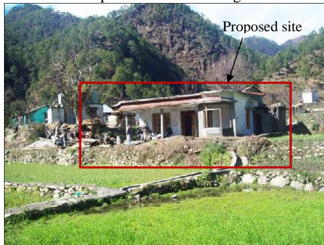
Uphill side view of the proposed site
