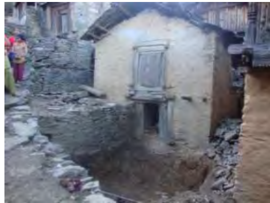
A side view from NE direction of the proposed site.
