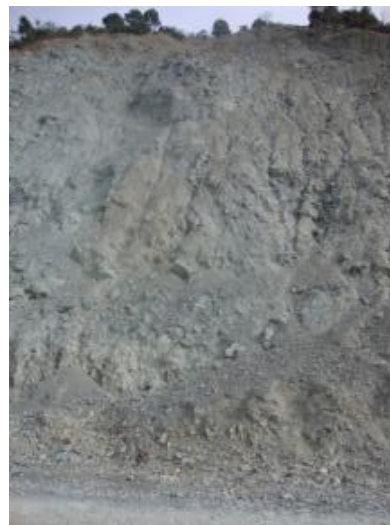
Landslide debris material.
